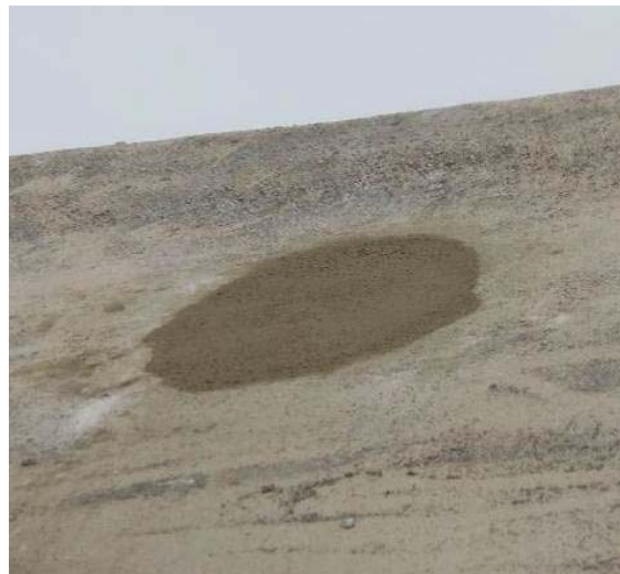
Figure 18. Lean Concrete Backfill on Ogee Anchor Holes
