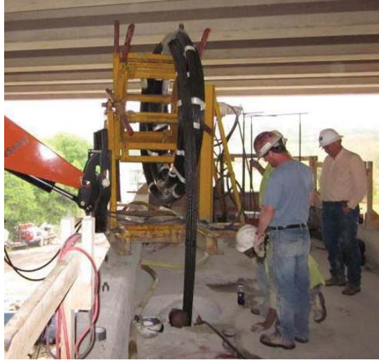
Figure 14. Installing Tendon with Uncoiler under the bridge
