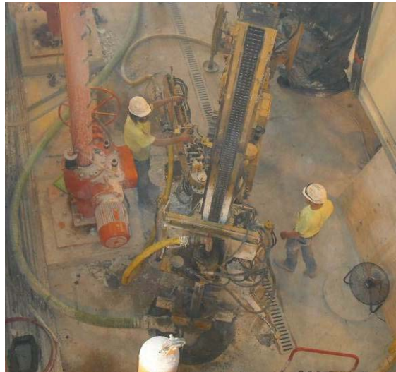
Figure 5. Limited Access Drill in Gatehouse
