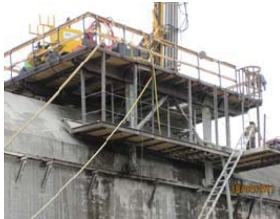
Figure 7. Moving Platform at Overflow Section
