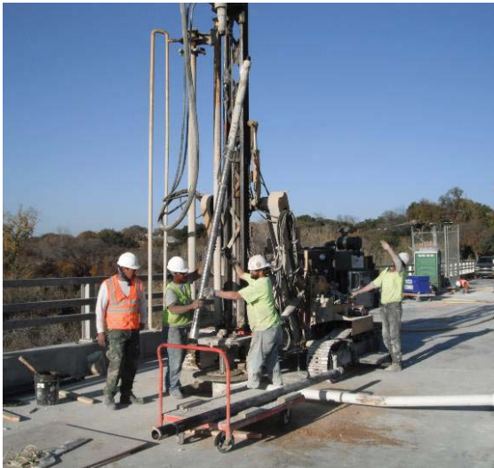
Figure 4. Drilling Rig on Left Abutment
