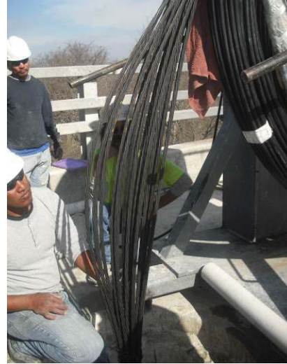
Figure 15. Strand Tendon Opening up During Uncoiling
