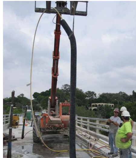
Figure 13. Corrugated 12 feet above grade for Leak Test
