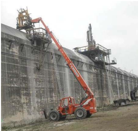
Figure 6. Access to Overflow Section
