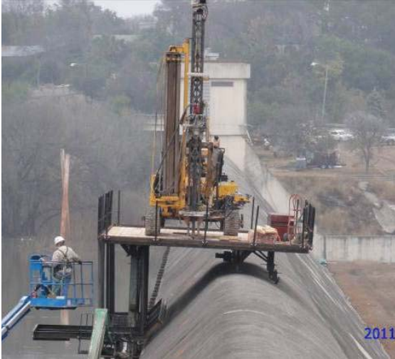
Figure 8. Rig on Moving Platform
