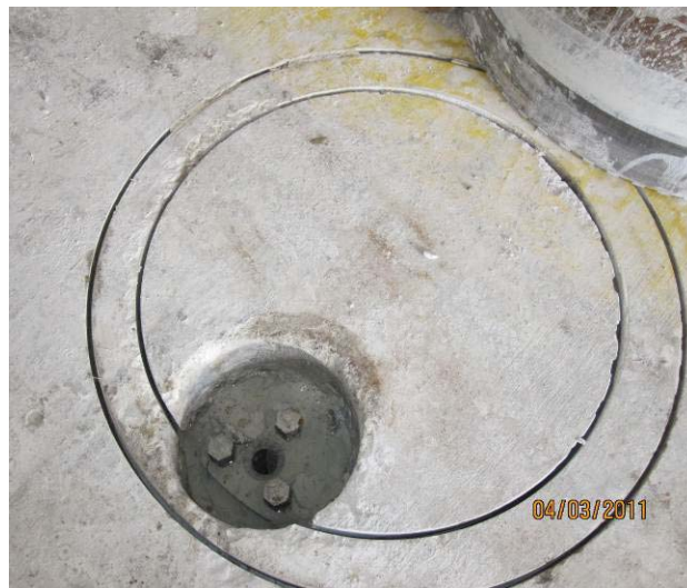
Figure 2. Pocket Overlap with Existing Anchors
